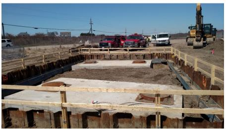
Vaults in a beach parking where two submarine cables come ashore. Post installation, only manhole covers are visible.
